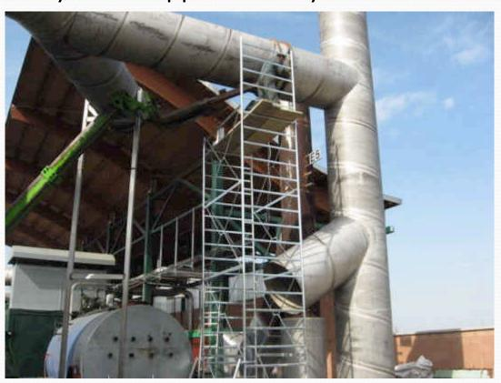
Erected the power plant in 2 locations using A305 & A316 stainless steel pipe material.
